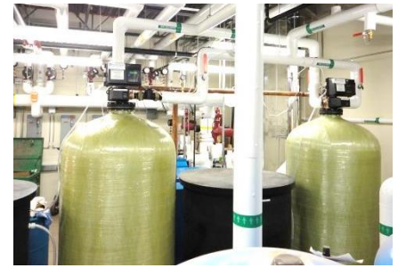
EDS3672-2-2900-TA softener operating in Twin-alternating configuration using 3200NXT controller
