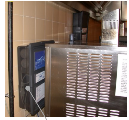
CORO wall mounted behind a combi-oven
