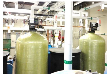
EDS3672-2-2900-TA softener operating in Twin-alternating configuration using 3200NXT controller
