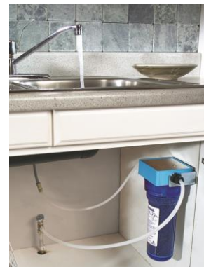
Install undersink on cold water pipe of existing kitchen faucet
